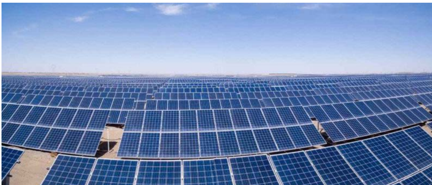
Figure 6: PV system in Jordan.
