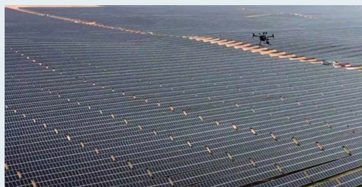
Figure 4: Inspection using drones.
